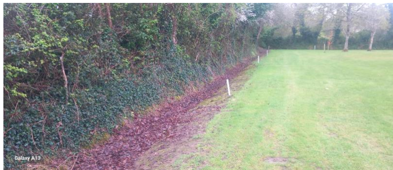
Treatment carried out to remove access vegetation
