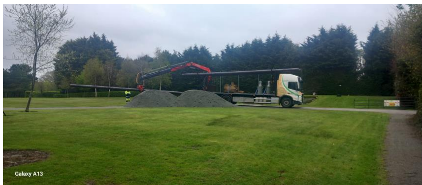
Pathway dust ready for spreading on paths throughout the golf course
