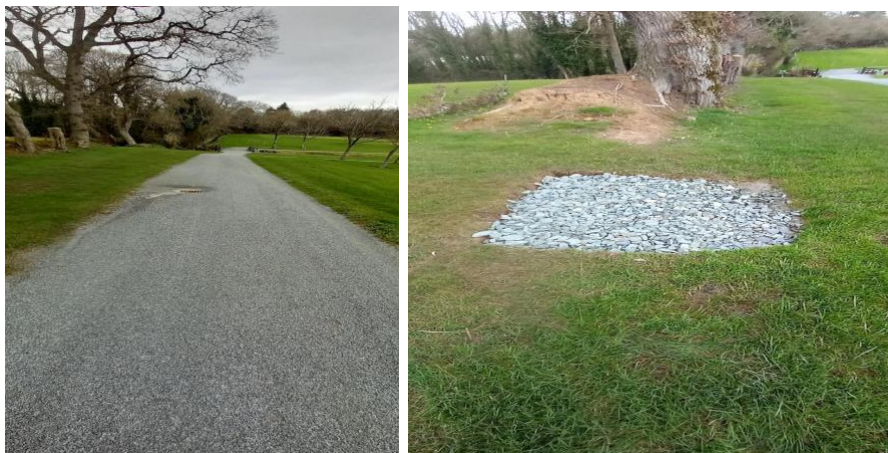
Pathway works leading to the maintenance yard and soak pit catching water off the land
