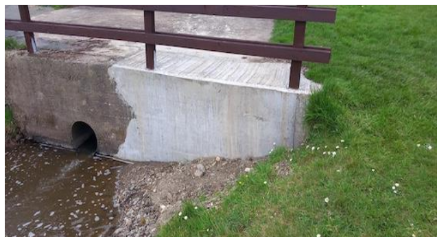
Bridge repair and painting of hand railings
