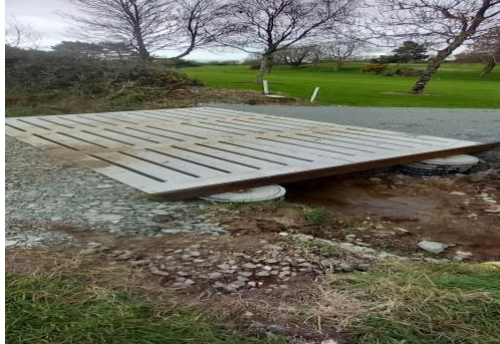
New bridge constructed with slatted concrete to allow water to enter into the ditch
