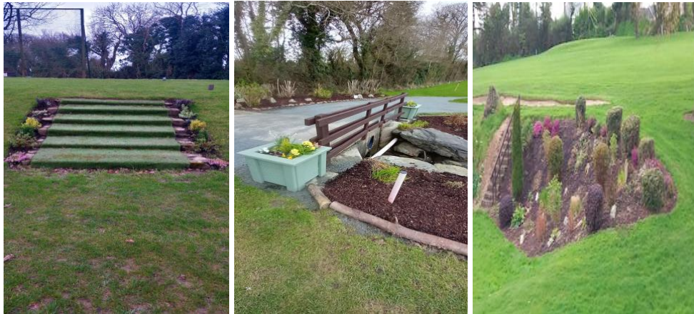
Landscape improvement works include bridge painting
